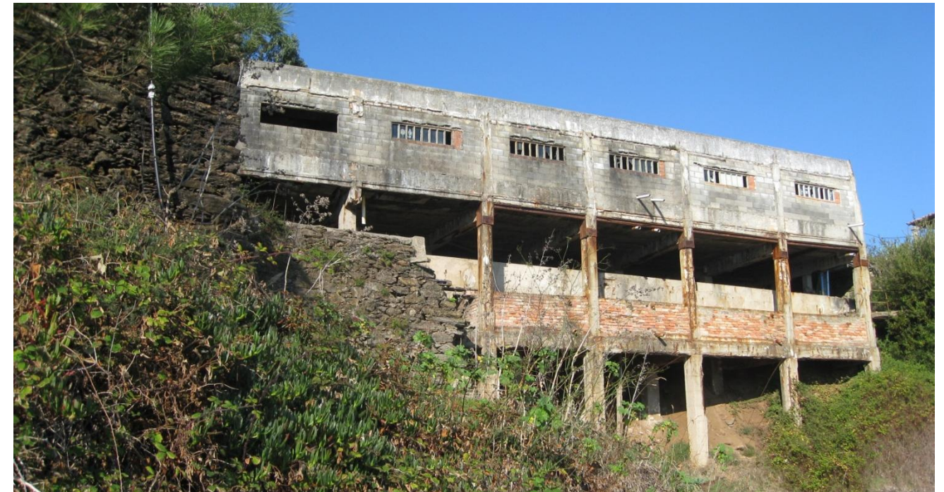
Nave a demoler en parcela catastral 4334641NG1943S0000QH
